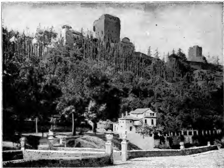
GENERAL VIEW OF THE ALHAMBRA
